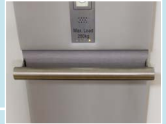
straight stainless steel hand rail
